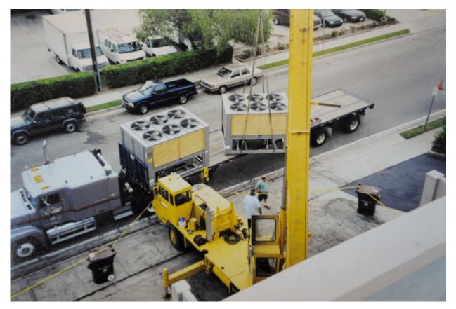
An example of one of the company's larger-scale projects. In this photo a crane lifts large air-conditioning units onto the roof of Midtown Plaza in Sarasota.
